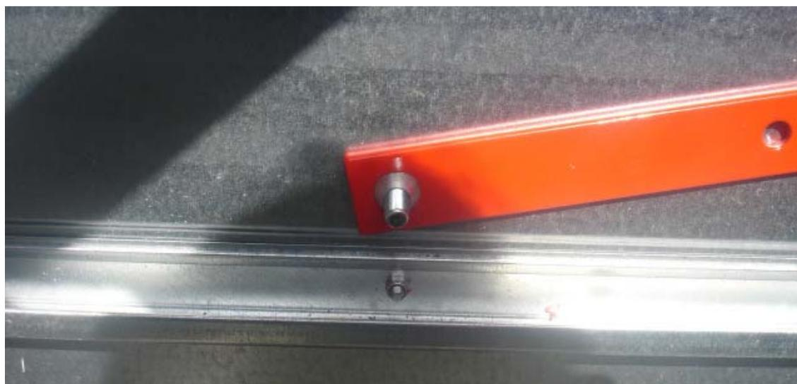
**12. Fit the anti-drill ball bearings to the bolt heads:** Go outside the shed and hammer one of the ball bearings supplied into the hexagonal head of each bolt. You may find the extra M8 x 50mm bolt is useful as a *punch* to reach the bolt heads – the end of the bolt has a slight dimple that will locate on the ball bearing. The ball bearings are a tight fit so it will take a smart hammer blow to drive them into the bolt heads. Be careful not to hit your fingers! ☺
