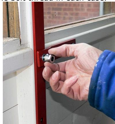
*Then fit a shear nut on top of the washer*
