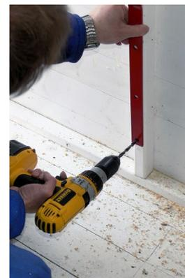
**15. Fit the side brace:** The last bolt will be fitted on the side brace, usually perpendicularly from the top extension bar. Another option would be with it fitted horizontally just above the floor, bolted to the bottom of the lower extension bar.
