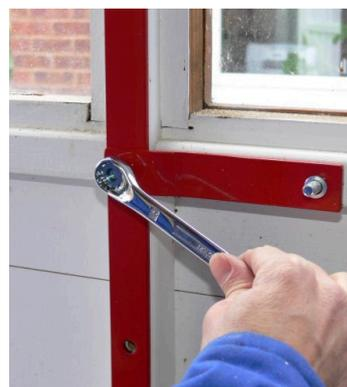
*Tightening shear nuts with a ring spanner...*
